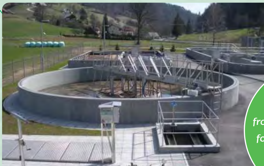
Waste water treatment plant Dobrna
