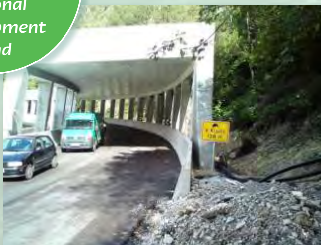
Finished reconstruction & building of gallery
