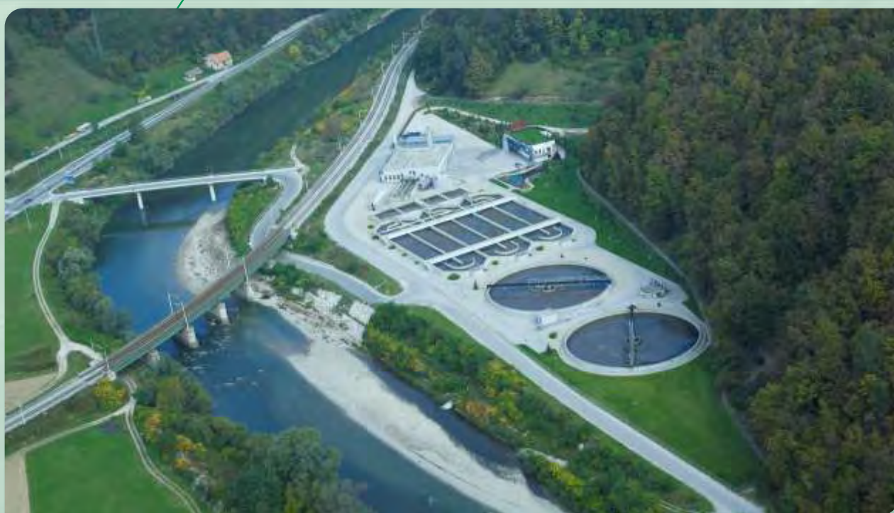
Waste-water treatment plant Celje
