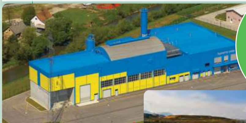
District heating plant
