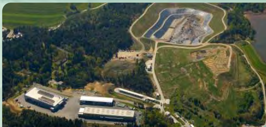
Landfill with other facilities
