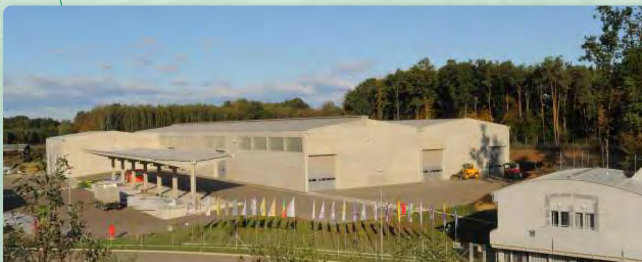
Mechanical treatment hall
